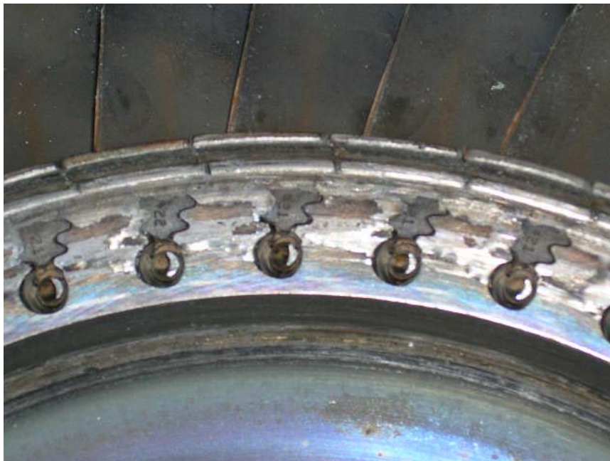
Photo No. 9 Compressor turbine downstream side detail.
